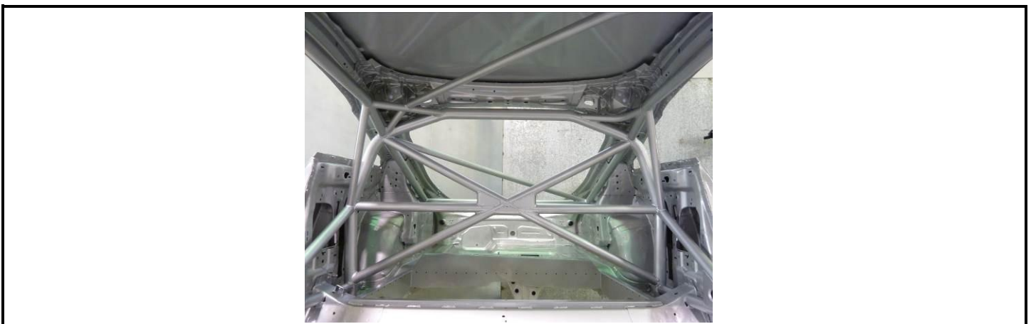
N1-6) Bare bodyshell – Roof seen from cockpit
